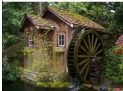
The water wheel of a mill for grinding grain into flour
